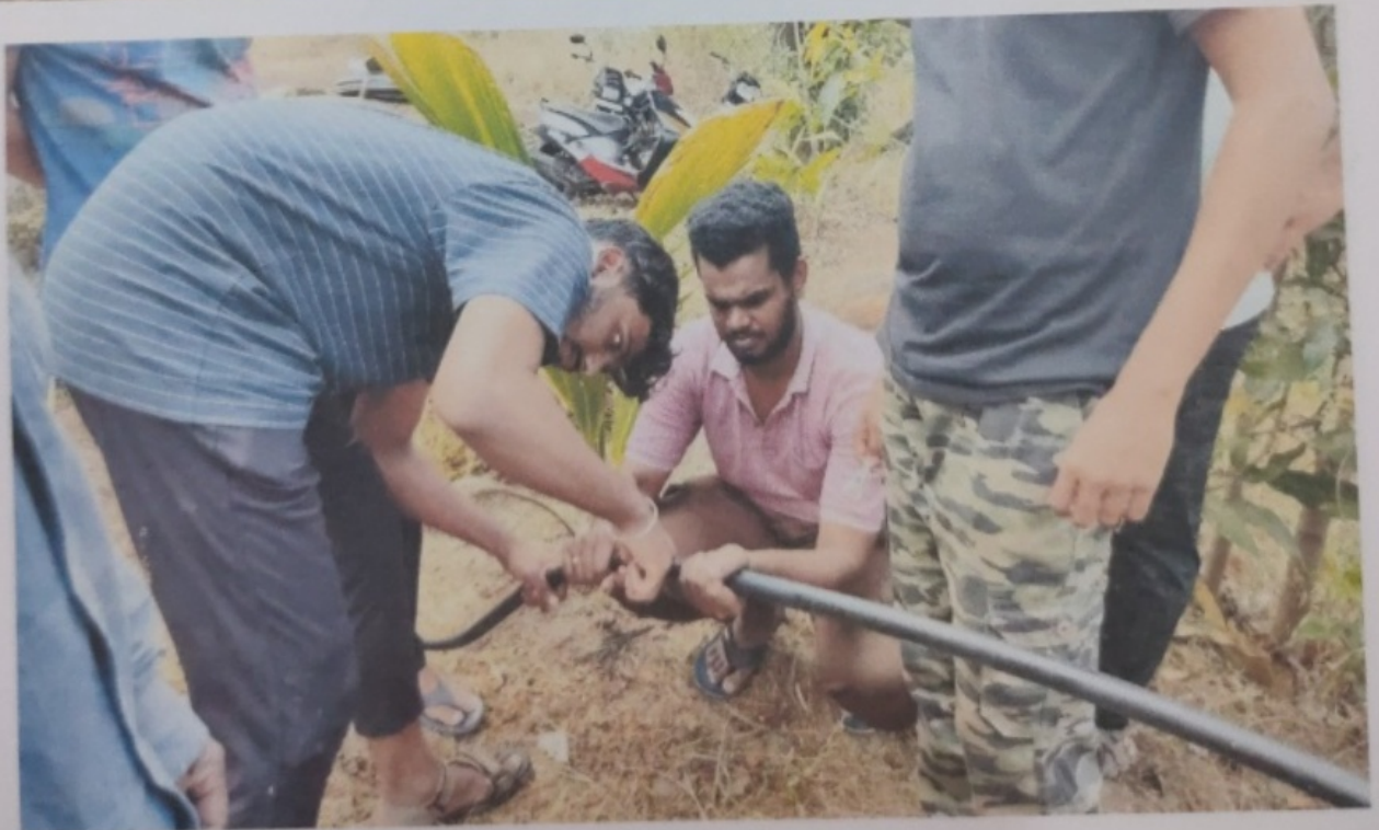
CAPTION: Fixing Bore Well Motor
