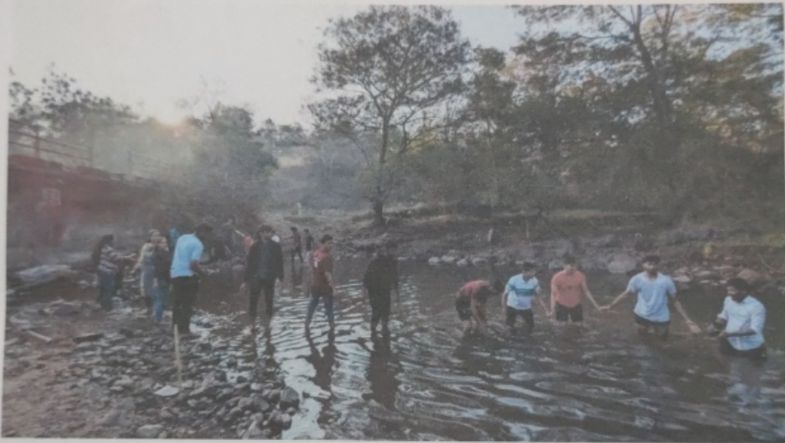
CAPTION: Increased the depth of the Pond and Blocked the Overflow
