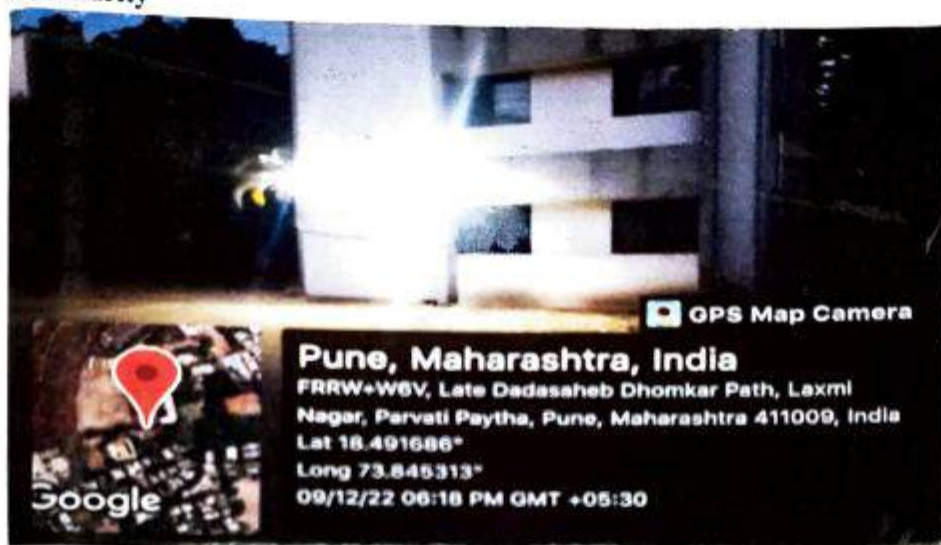
Photo: Street Lights in the Institute Campus.
