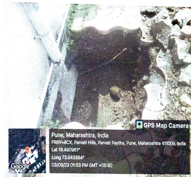
Figure C: Excavation for sockpit
