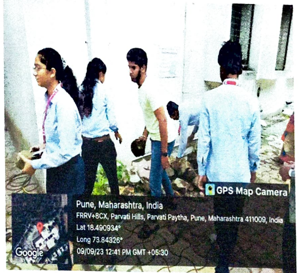
Figure D: Material Filling in sockpit
